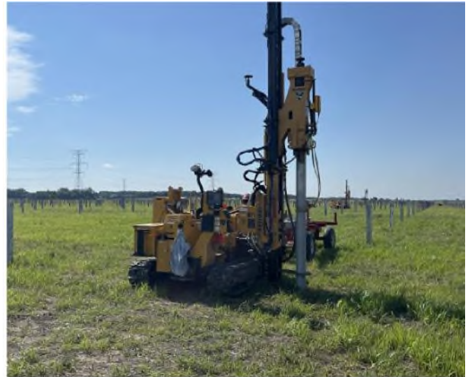
Pile drivin' Steel racking foundations are driven into Block 141 this summer.
